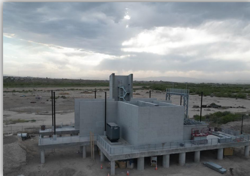
Figure 12 – Presidio Freight Rail Inspection Facility
